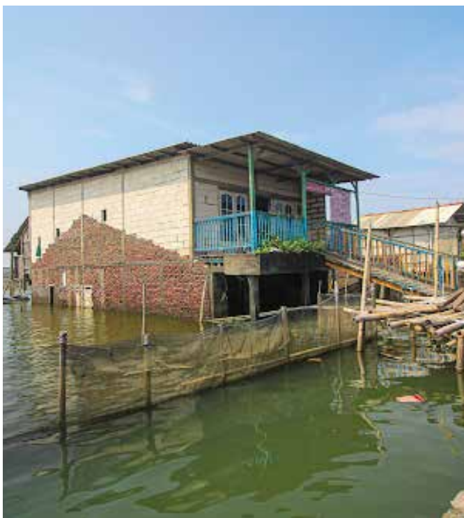
Figure 14. Up left and right: Damaged buildings in Sriwulan, Demak, Down-left: Sinking building in the coast of Sriwulan. Down-right: Raised buildings to adapt with land subsidence in Sriwulan, Demak. Source: Rafii Bisatya (2021)
