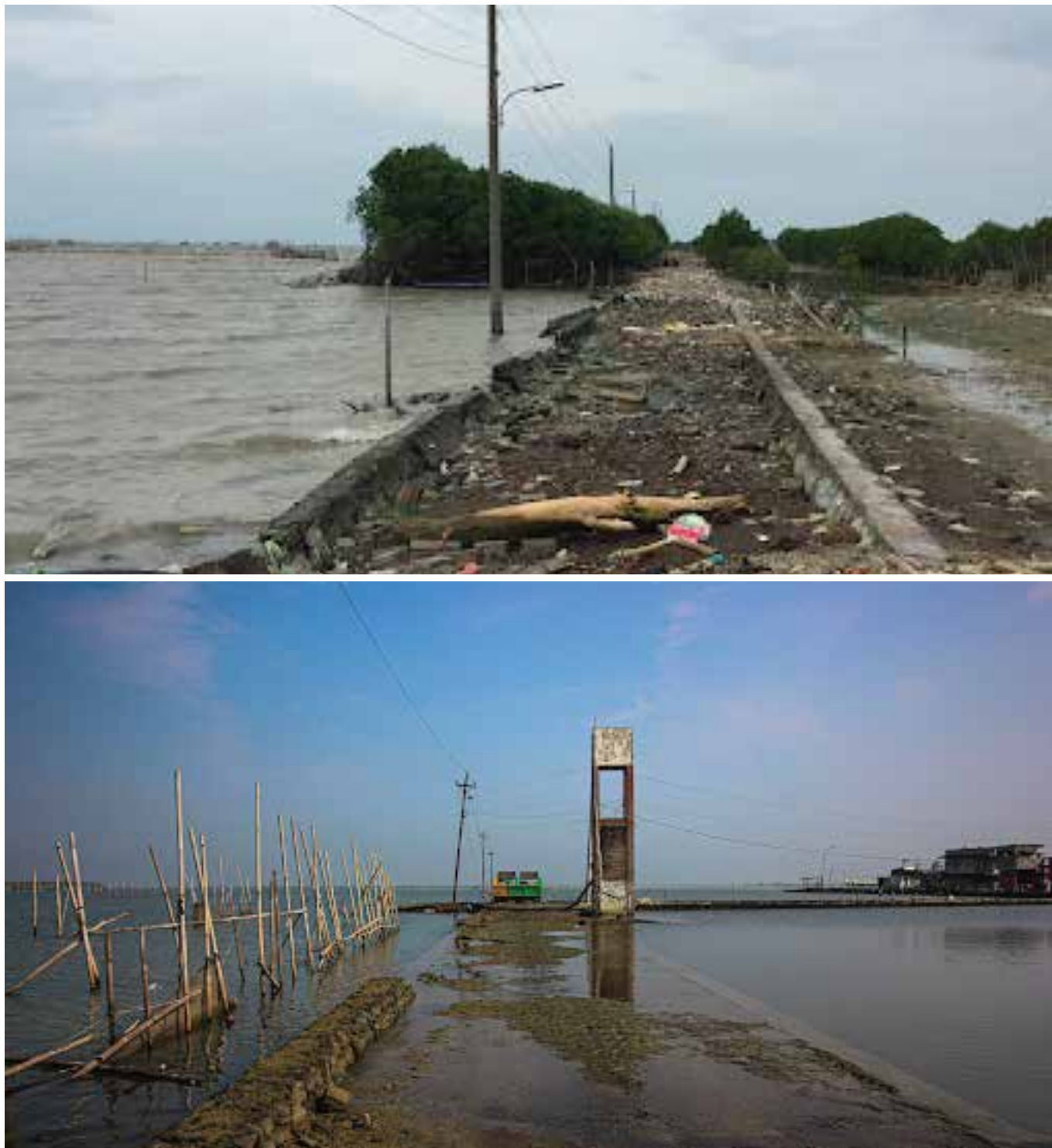
Figure 19. Damaged infrastructures in Sriwulan, Demak
