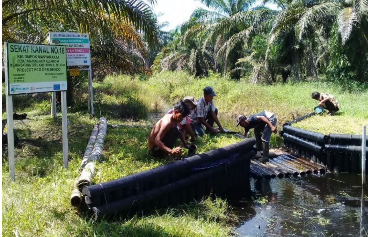
Community groups maintain canal blocks, which were built to contain the flow of water. Canal blocking functions to re-wet peat that has dried up due to drainage (canals are made), so that it is not prone to fire.
