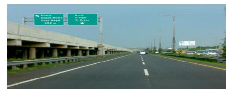
Figure 15. The toll road to the Soekarno-Hatta Air port in Jakarta has been raised up to 1.2 meter (left due to 'rhob' flood hits northern Jakarta more frequently after mangrove have been cleared (Photo: Ita Sualia, 2010)
