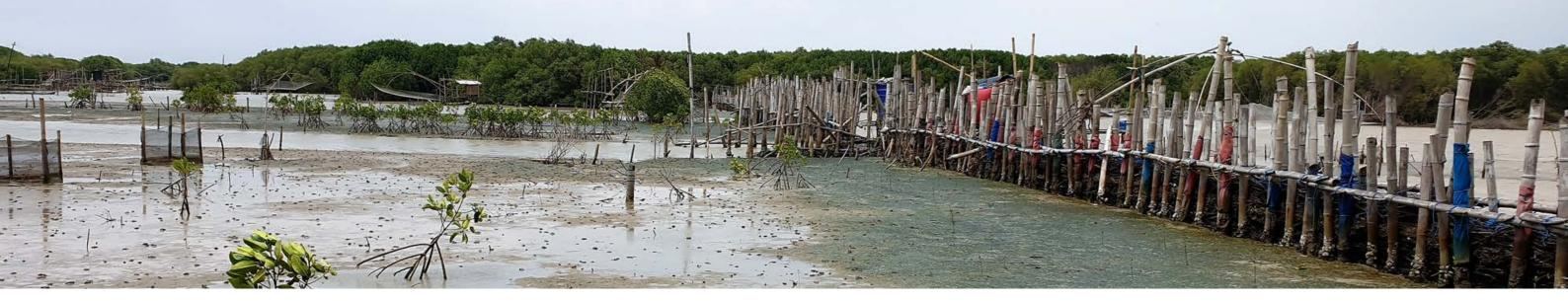
Figure 30: Increased sedimentation behind permeable structures in Demak ©Yus Rusila Noor
