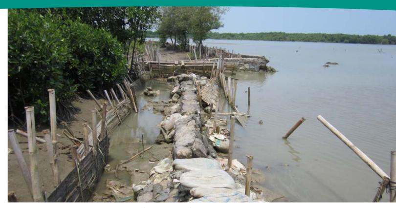
Figure 1: Failed seawall (Demak, Indonesia) © Bregje van Wesenbeeck
