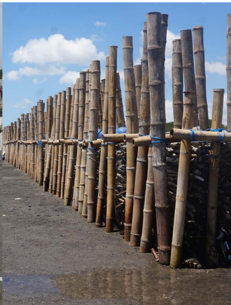
Figure 18: Permeable Structures constructed by the Indonesian Ministry of Marine Affairs and Fisheries (MMAF) in Lombok in 2019. ©MMAF
