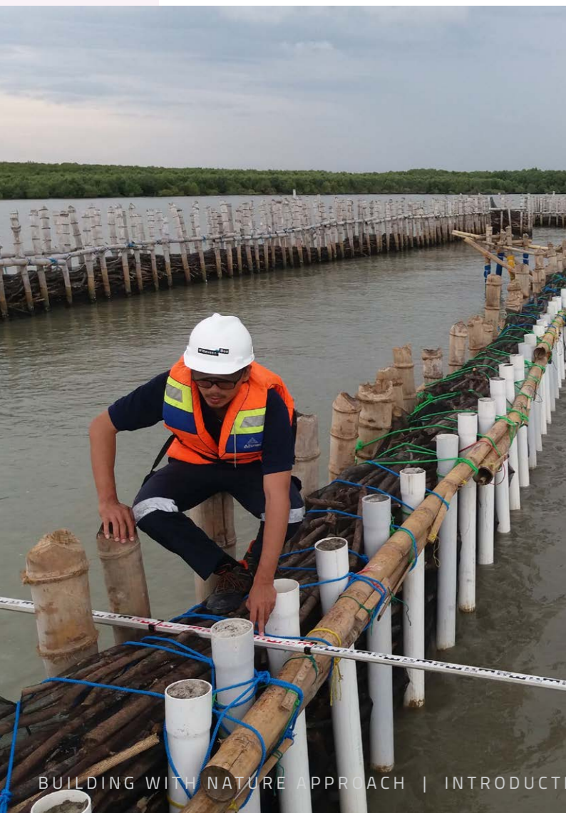
Figure 17: Monitoring of permeable structures in Demak. ©Witteveen+Bos
