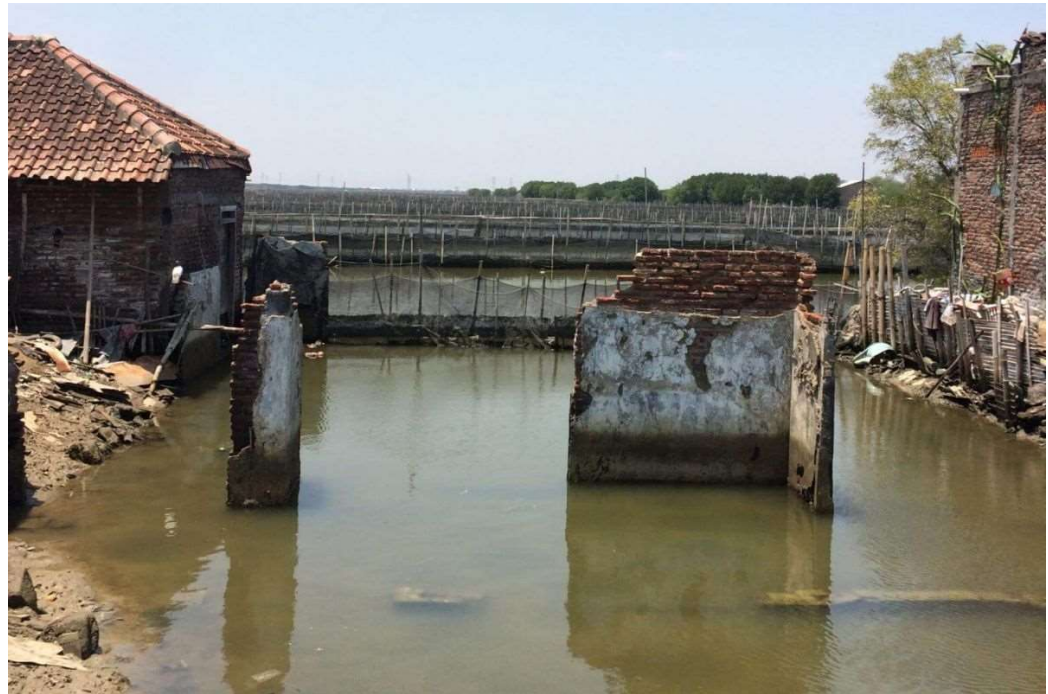
8.9: Evidence of land loss (Hutton, 2020)
