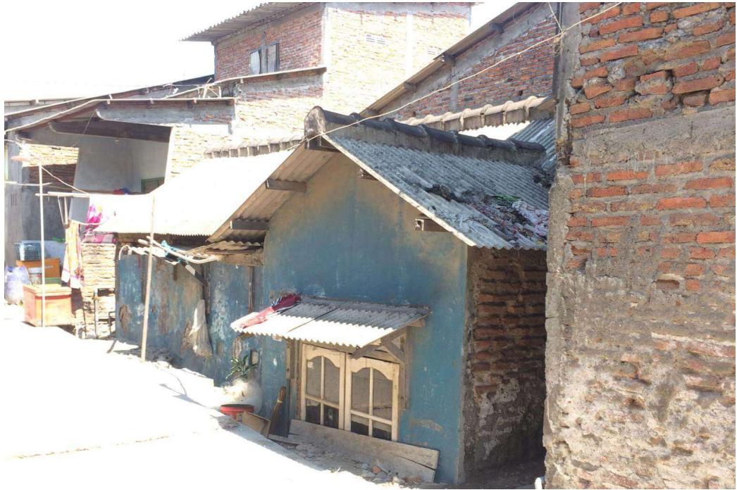
8.10: Evidence of elevated road in subsiding area (Hutton, 2020)
