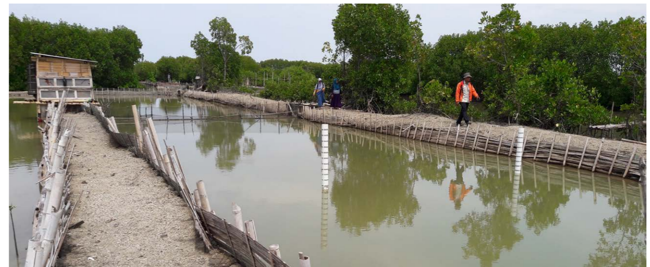
Figure 12: An image of the new dyke with the bamboo screens, attached to each other with iron wire, still in place, and the old river dyke in the background (© Roel Bosma)
