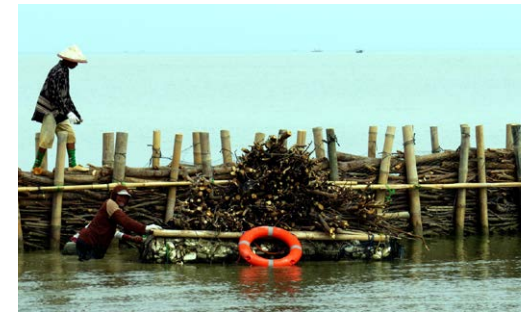
Figure 20. Floating transport and stockpiling © Bagus Maulana
