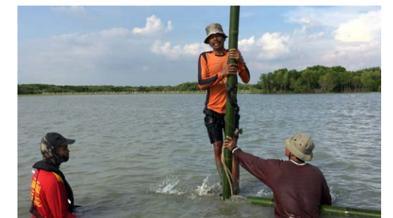
Figure 22. Manual installation of an individual pole © Deinar Santayana, Witteveen+Bos
