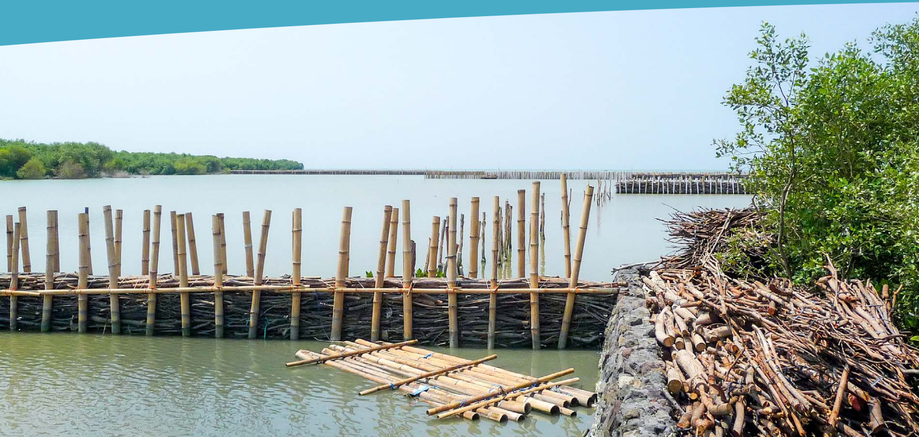
Figure 1. Permeable structures in Timbulloko (Demak, Indonesia) © Tom Wilms, Witteveen+Bos
