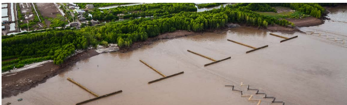
Figure A.5 – Restoration of eroded floodplains using bamboo T-fences in Bac Lieu Province (Mekong Delta, Viet Nam). © Cong Ly and G.E. Wind 2013.
