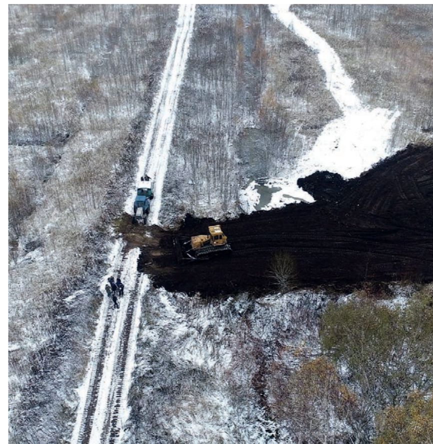
Tver oblast peatland in Russia during winter restoration activities.
