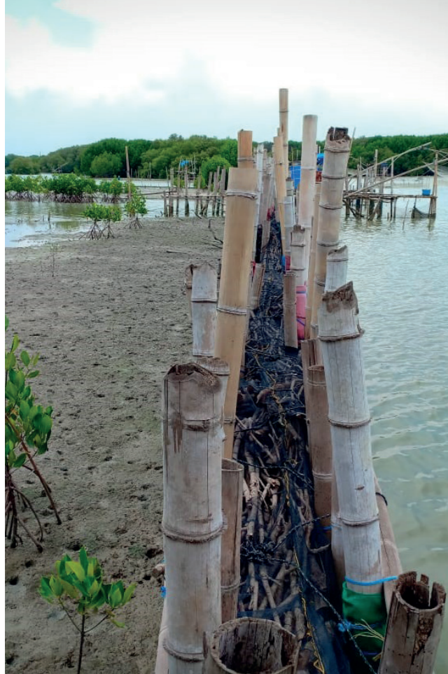
Permeable structure that traps sediment to stabilise the coastline at Bogorame Timbulsloko village, Java.
