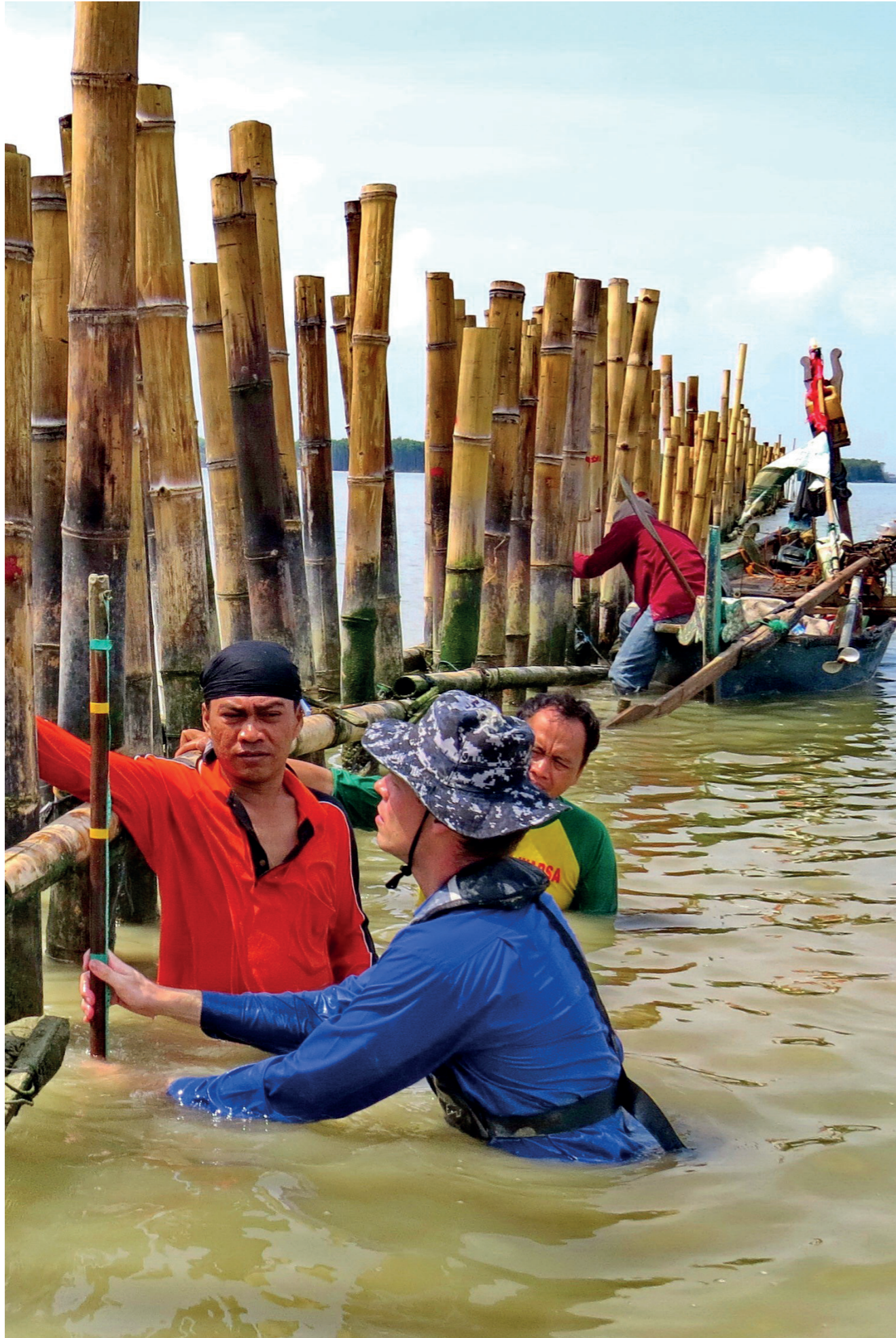
Community establishes permeable structure to catch sediment to let mangroves grow back naturally.
