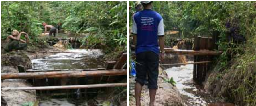
Illustration 75. System of opening and closing temporary blocks in ditches near the Merang River. Left: Closed block with a log being floated down. Right: Open block so the log can float by. (Photograph: Suryadiputra, June 2004)
