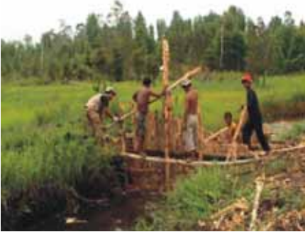
Illustration 81. Installing Upright Supports
