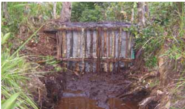
Illustration 73. Construction of Block in Sami Canal after Completion (Documentation: WWF-Indonesia/Eko Manjela, 2004)
