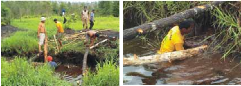
Illustration 79. Installing Top and Bottom Cross Supports
