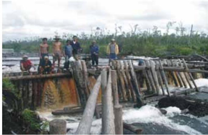
Illustration 32. Belangiran bracing poles at the back of a block (Photograph: Suryadiputra 2004).
