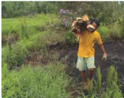
Illustration 78. Collection of materials for constructing the dam.
