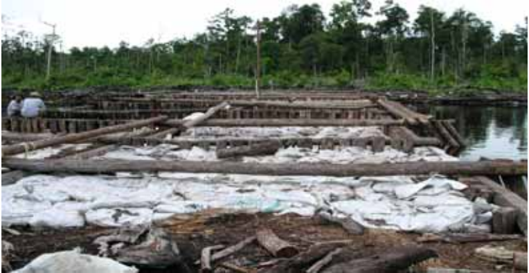
Illustration 34. Block SPP-SPU7 after being filled with soil sacks (Photograph: Suryadiputra 2004).
