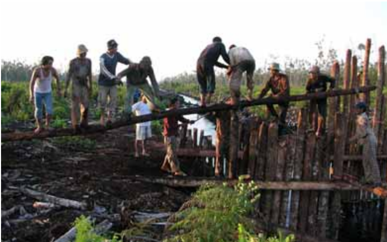
Illustration 31. Workers jump up and down on horizontal log (Photograph: Suryadiputra 2004).
