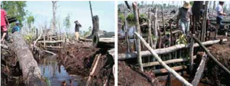
Illustration 51. Constructing the Block (Photograph: Suryadiputra, 2004).
