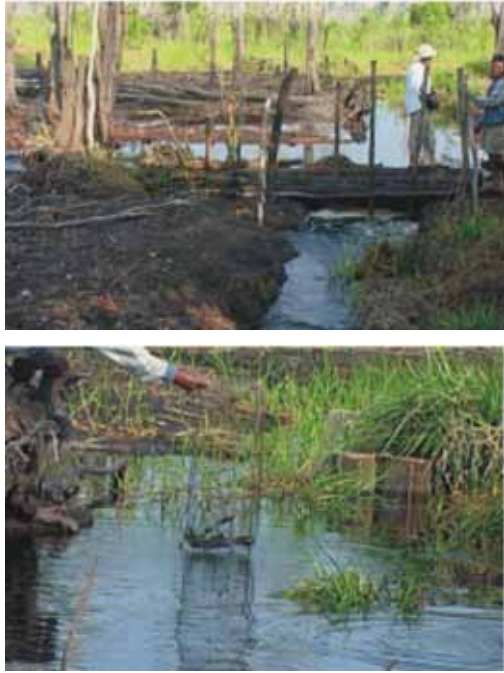
Illustration 56. Difference in water level above and below the block (top) and fishing activity in the blocked section of Ramunia ditch (bottom) (Photograph: Suryadiputra, June 2004).
