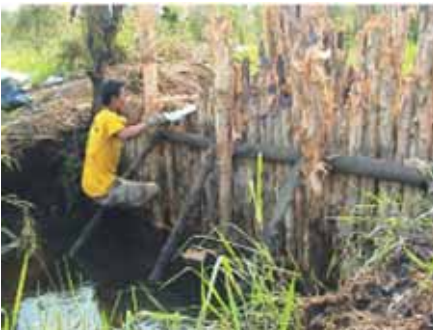
Illustration 82. Inserting Supporting Posts
