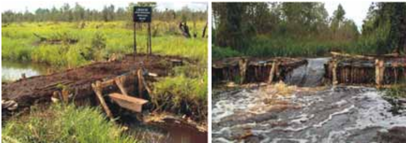
Illustration 85. The spillway was built in the middle of the block
