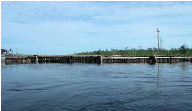
Illustration 35. Block SPI-1 No1. after completion (Photograph: Alue Dohong 2004).
